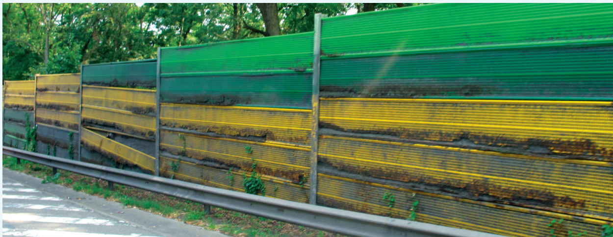
Image: © SPW Mobility and Infrastructures.
